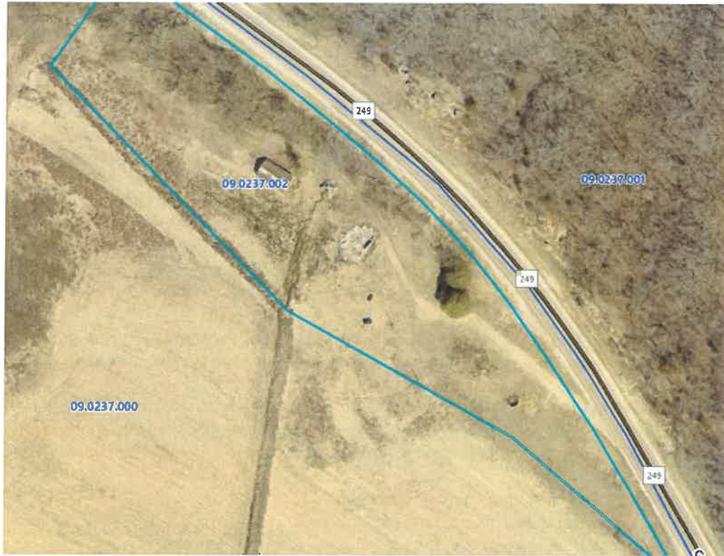
Figure 2. Aerial imagery from 2023 after the original dwelling was removed.
